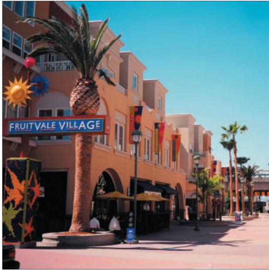
Oakland's Fruitvale Village was built as a TOD and is intended to revitalize its adjacent neighborhoods.
