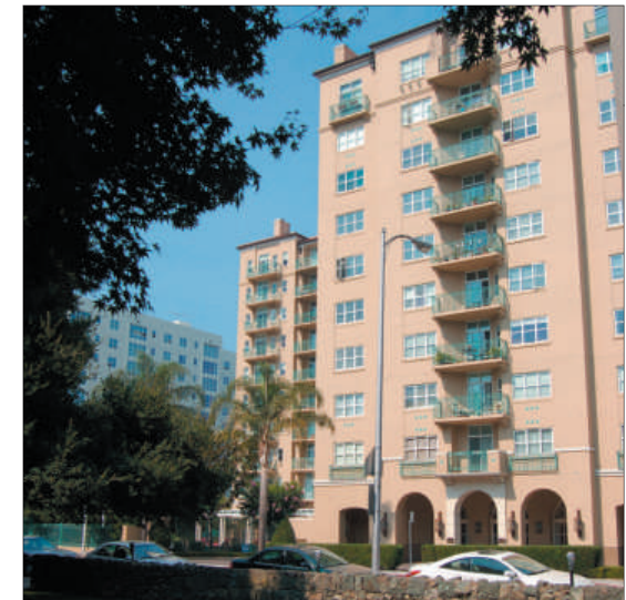
TOD-BART Area Mixed-Use - 100 units/acre. (San Mateo, CA)
