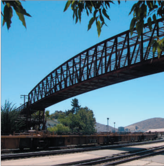
A pedestrian bridge crossing heavily-used railroad tracks connects a residential neighborhood to downtown San Luis Obispo.
