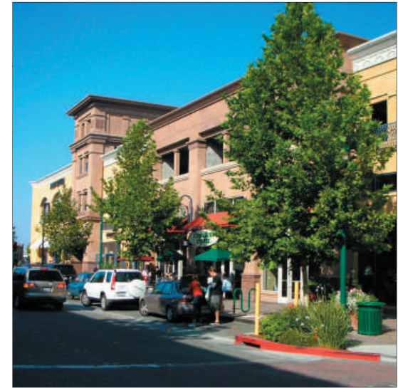
Downtown parking structure integrated into retail building design. (Walnut Creek, CA)
