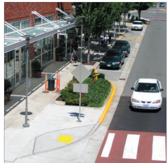
Corner bulbouts reduce the intersection crossing distance for pedestrians and provide additional streetscape amenity opportunities within the pedestrian zone.
