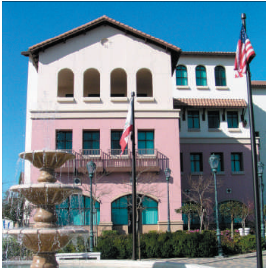
Office Mixed-Use - Creekside Plaza in San Leandro.
