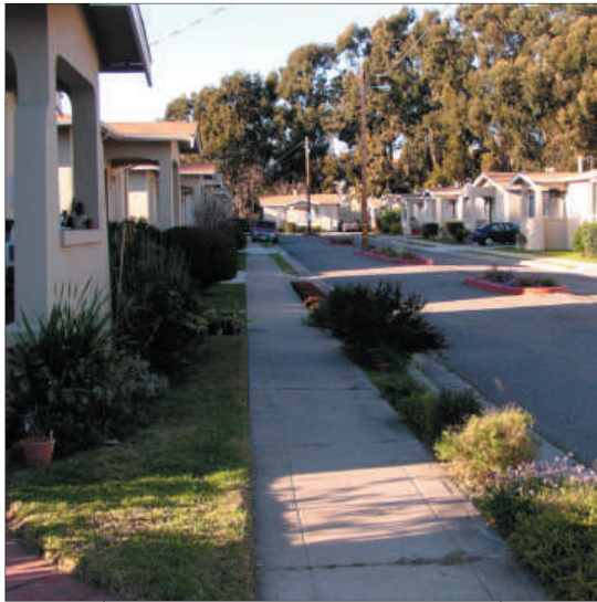
Residential Conservation District - Single-family residential neighborhood at Chumalia Street and Cecelia Court.
